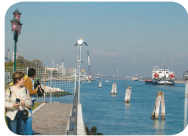
SL-125-C lanterns installed at marina, Venice, Italy
